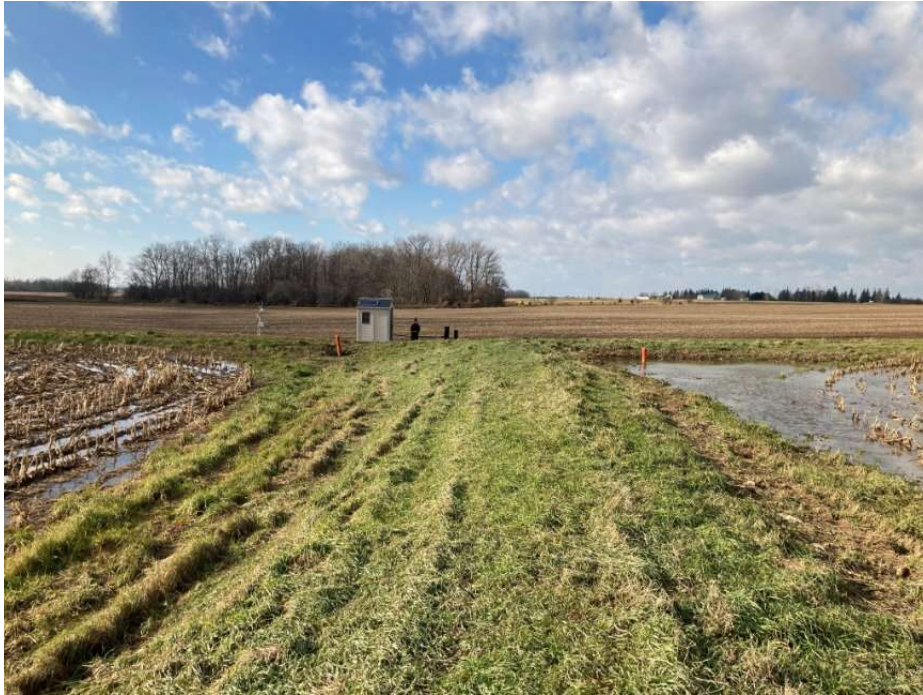
Figure 9. Photo of T-shaped berm separating the two monitored catchments at the North Kettle EOF.
