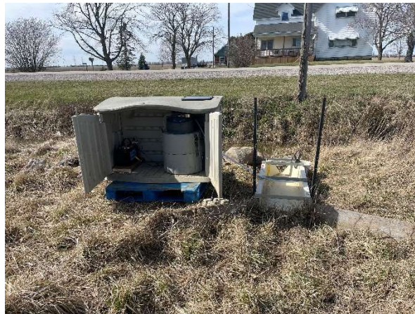
Figure 5. Merlin A's flume newly installed permanent enclosure with a solar panel.
