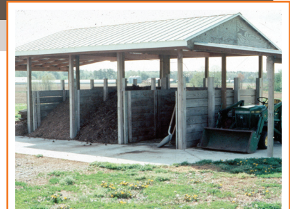
A roofed compost site will divert clean water from mixing with compost and producing runoff.
