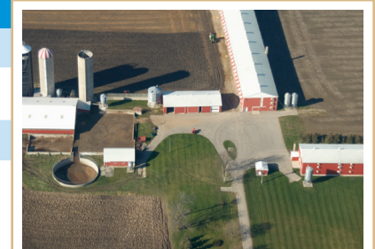
All runoff from this walled yard is captured in a liquid storage tank.
