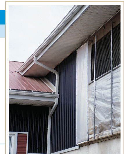
A properly designed eavestrough system will direct clean water away from storage or yard areas.
