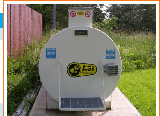
Evaluate condition of existing fuel storage tanks and maintain the corrosion protection.
