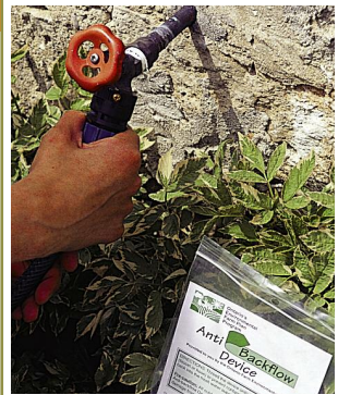
Anti-backflow devices should be attached to any faucet that supplies water for pesticide application.
