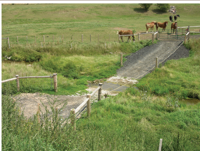
A fenced, bed-level crossing will manage livestock impact on the watercourse while providing access to pastures.
