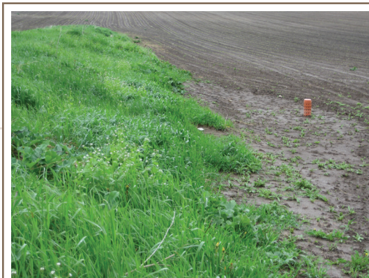
Surface inlets move excess surface water on cropland to subsurface drainage systems in a controlled manner that reduces soil loss.
