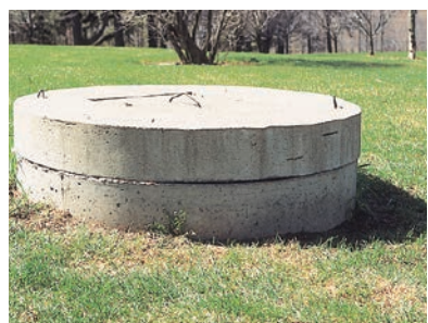
Bored/dug wells with concrete lids are considered vented.
