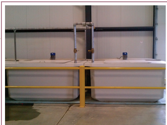
Locate stock tanks in areas with minimal or no traffic, and protect them from accidental impact.
