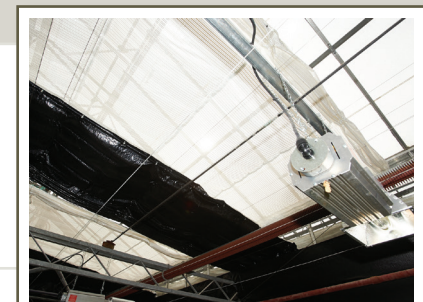
The use of blackout curtains on this greenhouse helps to reduce the offsite impact of grow lights.
