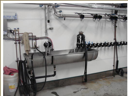
By using an energy conservation sink, you can reduce water use by as much as 45%.
