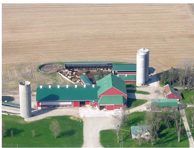
Relining silo walls helps to seal in seepage and maintain structural integrity.
